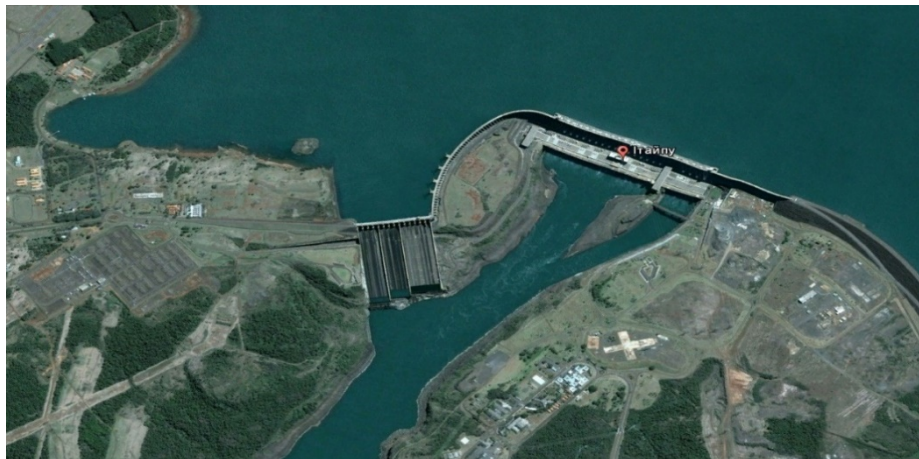
Fig. 3. Satellite image of the Itaipu hydroelectric station on the border of Brazil and Paraguay. Obtained using Google Earth Geosource
