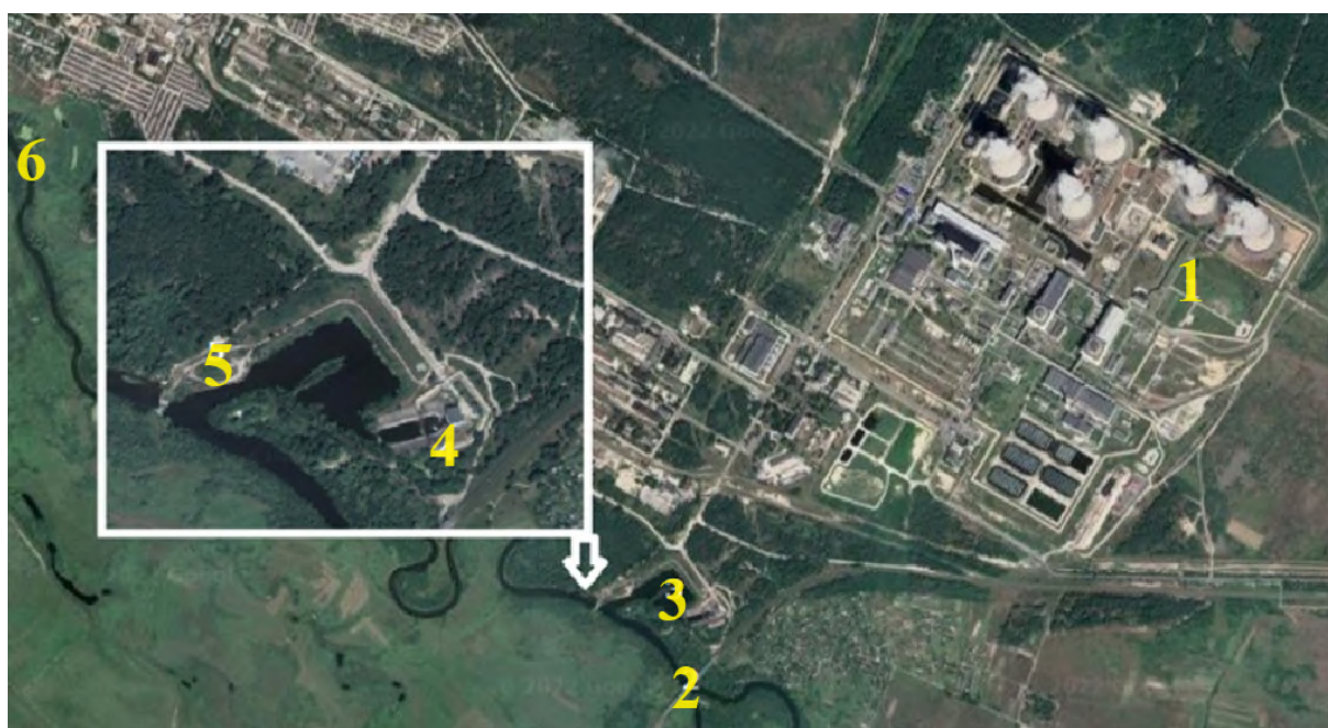
Figure 1. The scheme Styr River water intake and discharge for the RNPP (1 – site of the RNPP; 2 – Styr River; 3, 4 – water intake; 5 – return water discharge; 6 – hydrological post).
