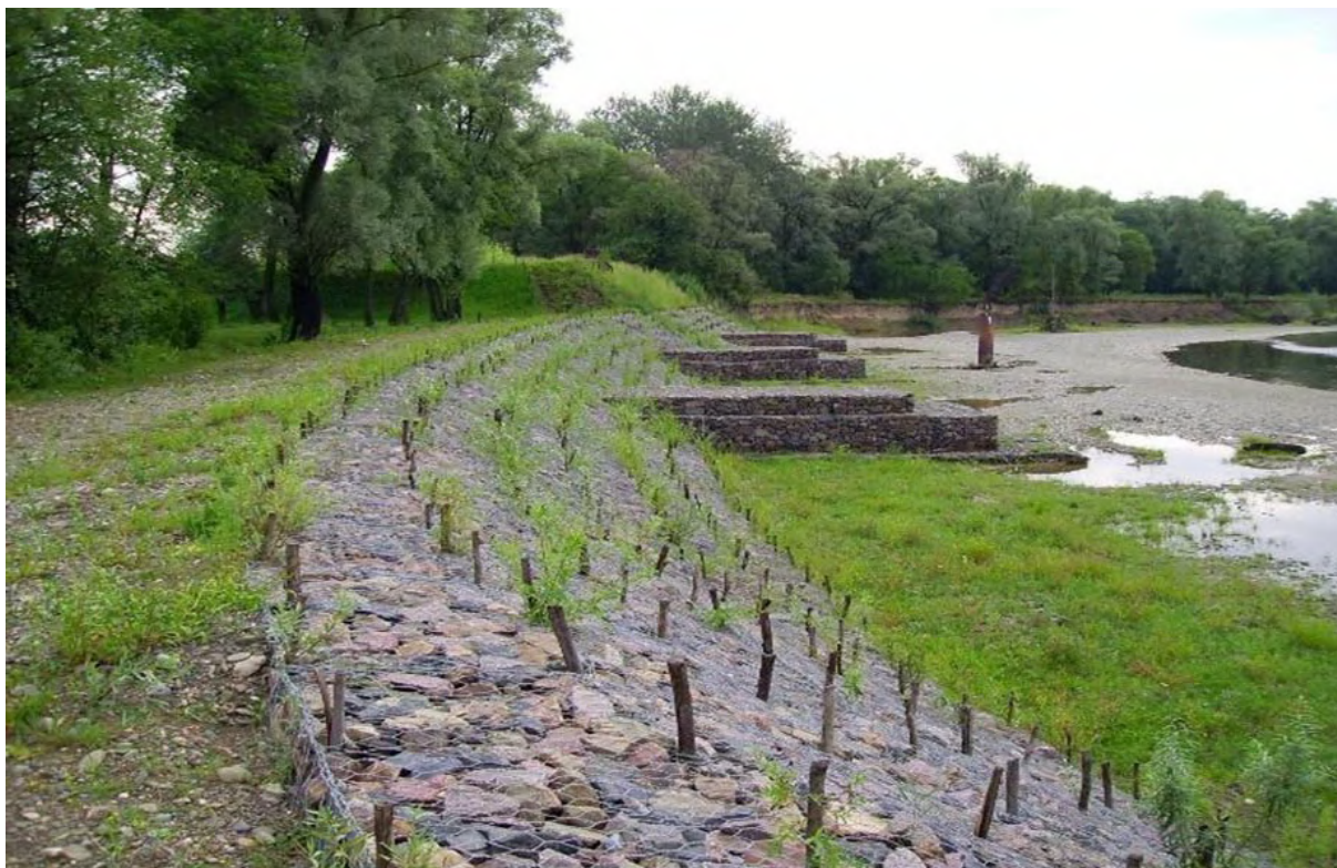
Figure 2. System of short fortifications of the river Siret, Storozhynets district, Chernivtsi region.
