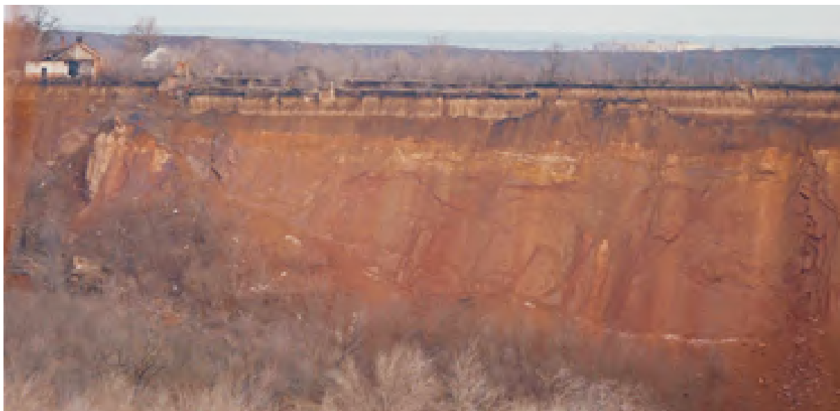
Figure 2. Land collapse with the destruction of housing (photo by Archil Svanidze).
