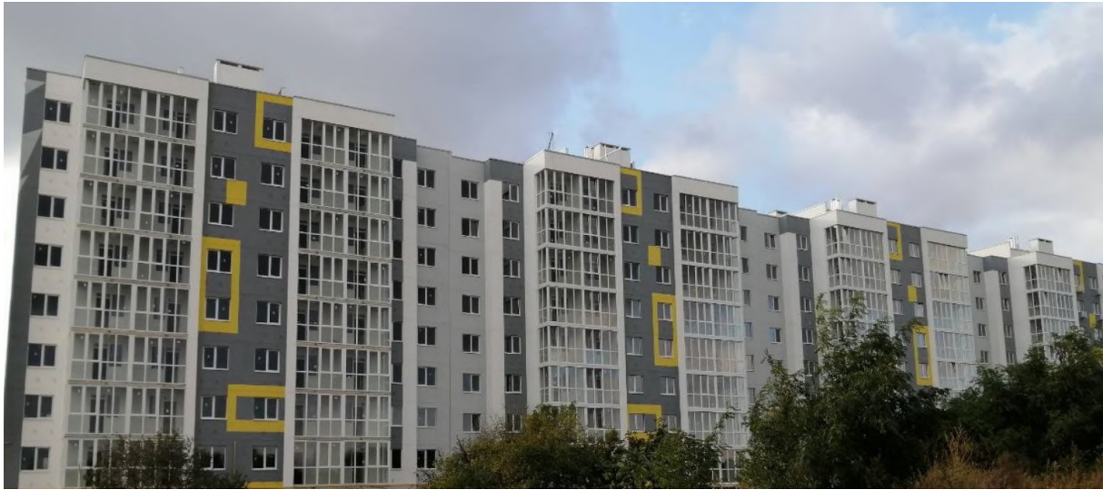
Figure 1. One of the new buildings of precast flat plate frame structural system in Poltava.
