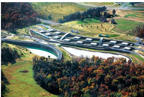
Fig. 27. General view of the Howard Hughes Medical Institute, Virginia, USA. Source: https://www.e-architect.com/america/howard-hughes-medical-institute
