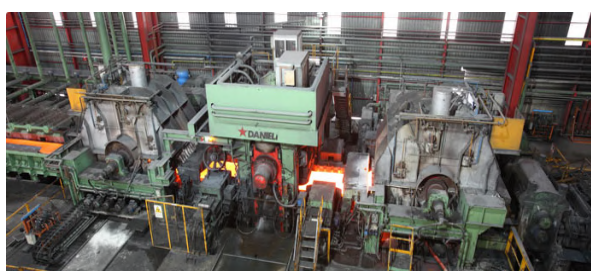
Fig. 2. Finishing stand of the Steckel mill 1780/quarto with furnace coilers.
