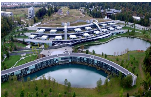
Fig. 26. General view of the Howard Hughes Medical Institute, Virginia, USA. Source: https://www.e-architect.com/america/howard-hughes-medical-institute
