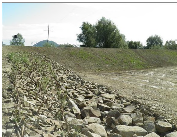
Fig. 7. Reconstructed protective dam to protect the city of Khust from floods (2011) [21].
