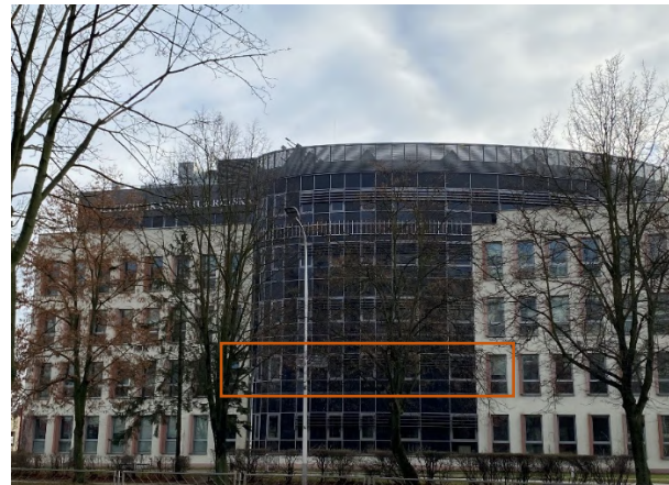
Fig. 1. Photo of “Energis” building and selected room where the test was performed.
