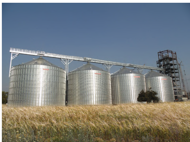
Fig. 2. Arrangement of silos in a row at the warehouse of the enterprise.
