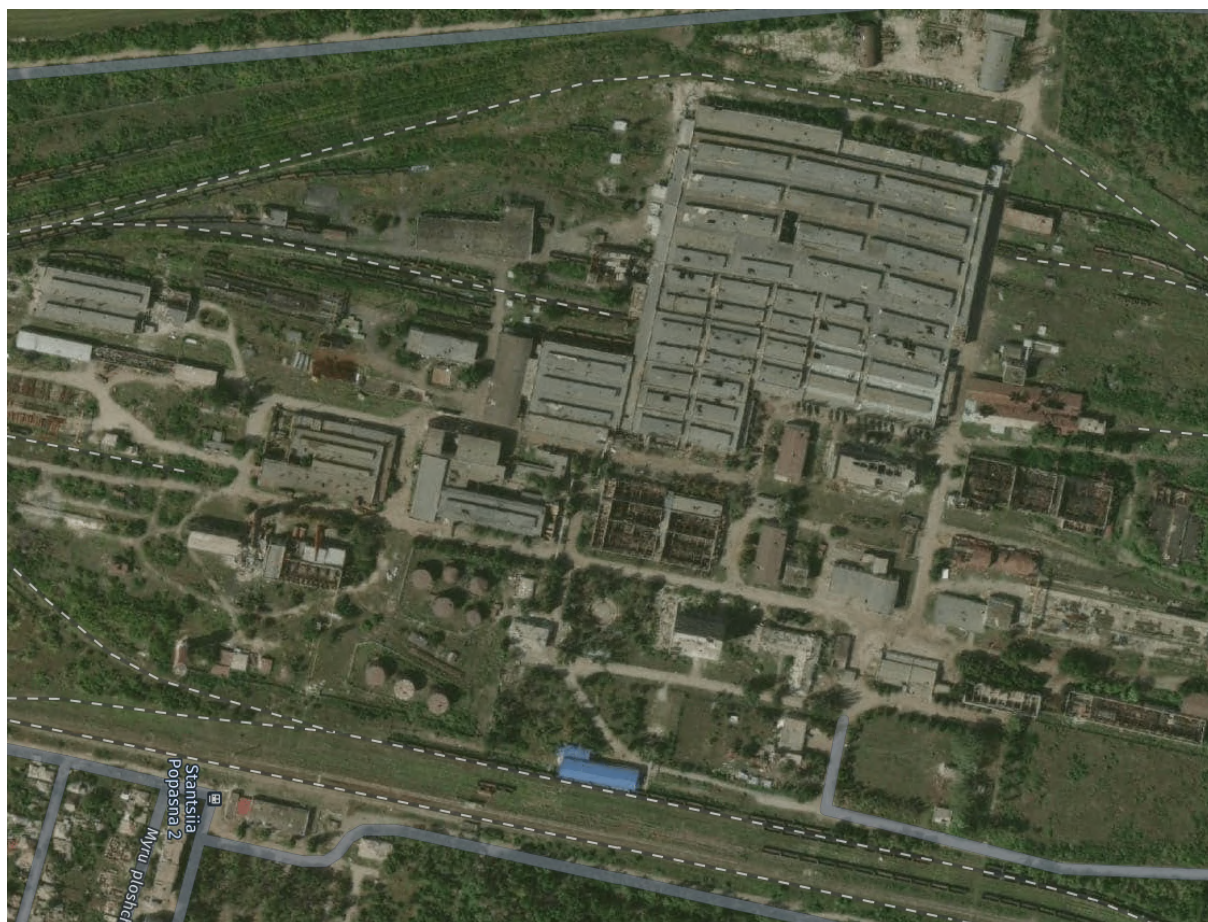
Figure 4. Satellite image of the damaged locomotive bay and wagon depot in the city of Popasna, Luhansk region [15].
