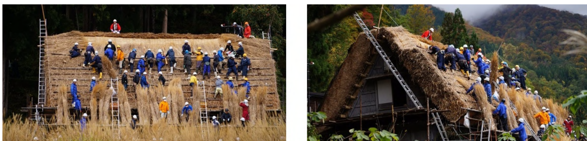
Figure 3. The roof replacement in Shirakawa village Ogimachi.
